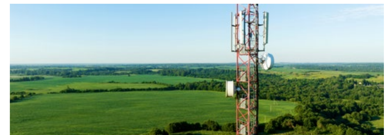
Vantage Towers, telecommunications towers Infrastructure | Europe | Partner: Global Infrastructure Partners
