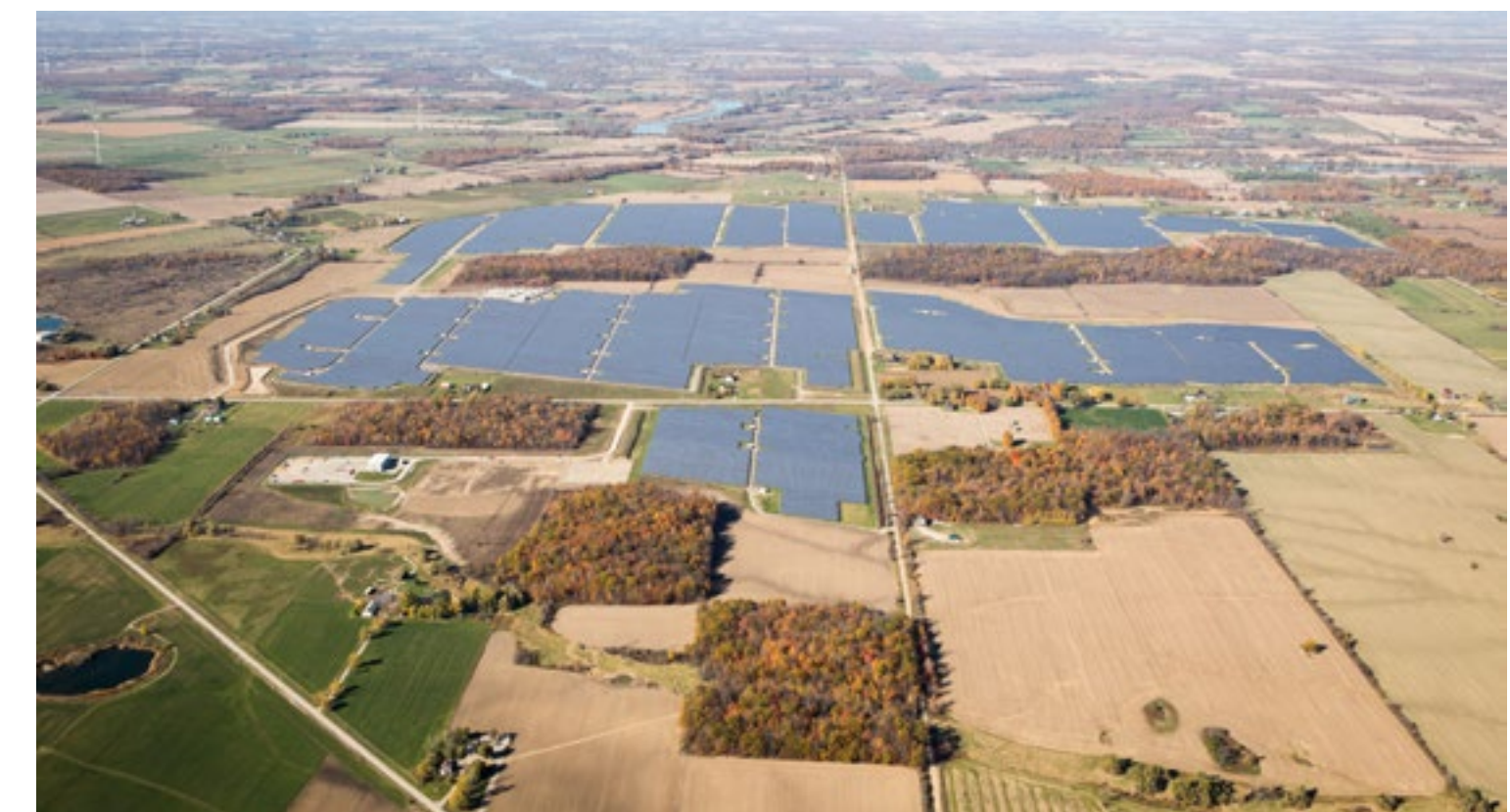
Haldimand Solar Project Infrastructure | Ontario, Canada | Partner : Connor, Clark & Lunn Infrastructure
