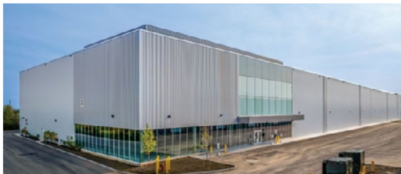
3540 and 3560 Wycroft Road, distribution centre Real estate | Ontario, Canada | Partner: Carttera
